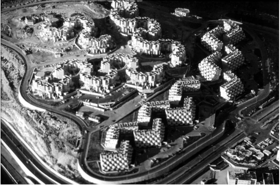
Figure 27.4 Zvi Hecker, Ramot Housing II, Jerusalem, Israel, 1978–1985 (aerial view). Courtesy of Zvi Hecker.
