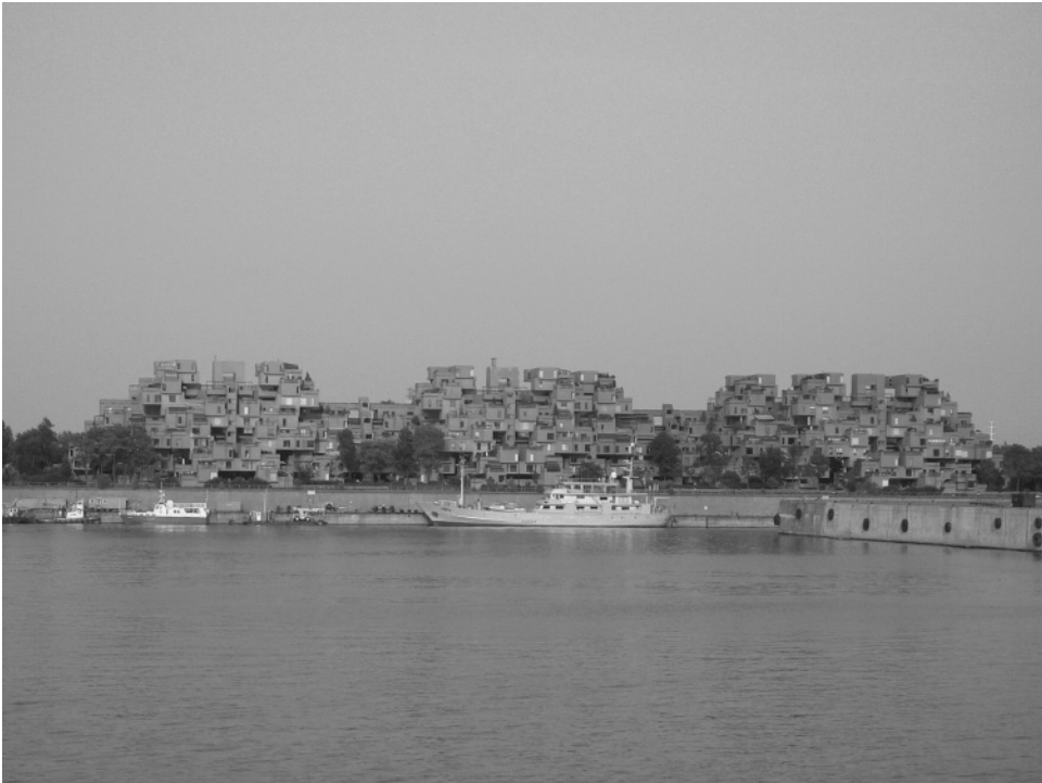
Figure 27.3 Moshe Safdie’s Habitat 1967 Housing Complex, Montreal. (Photography by Anthony Vidler)
